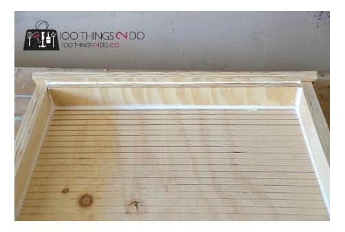
Before attaching your top plates, run another strip of caulking along the side and inner roof pieces and press tightly. Screw into place using  $1 \frac{1}{2}''$  galvanized screws while the caulking is still wet (it will give it a better seal). Line your front upper along the inner roof piece and screw down from the front. Before attaching your front lower piece, leave an opening between the boards that is  $\frac{1}{4}''$  to  $\frac{1}{2}''$  for ventilation.
