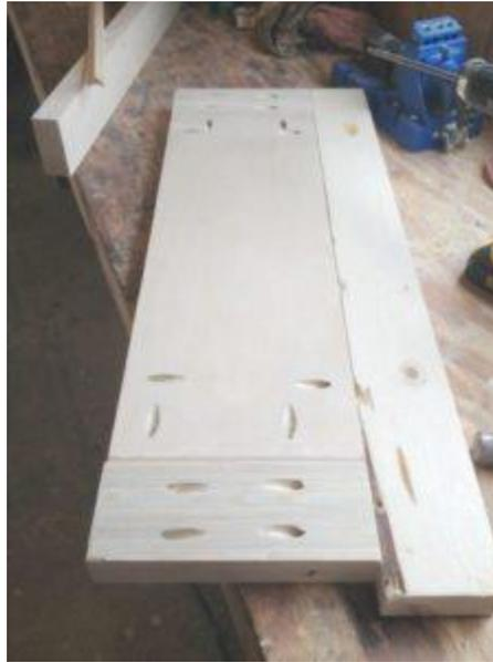
Lastly, I attached the last 2x4 to complete the two side panels attached using pocket holes and screws.
